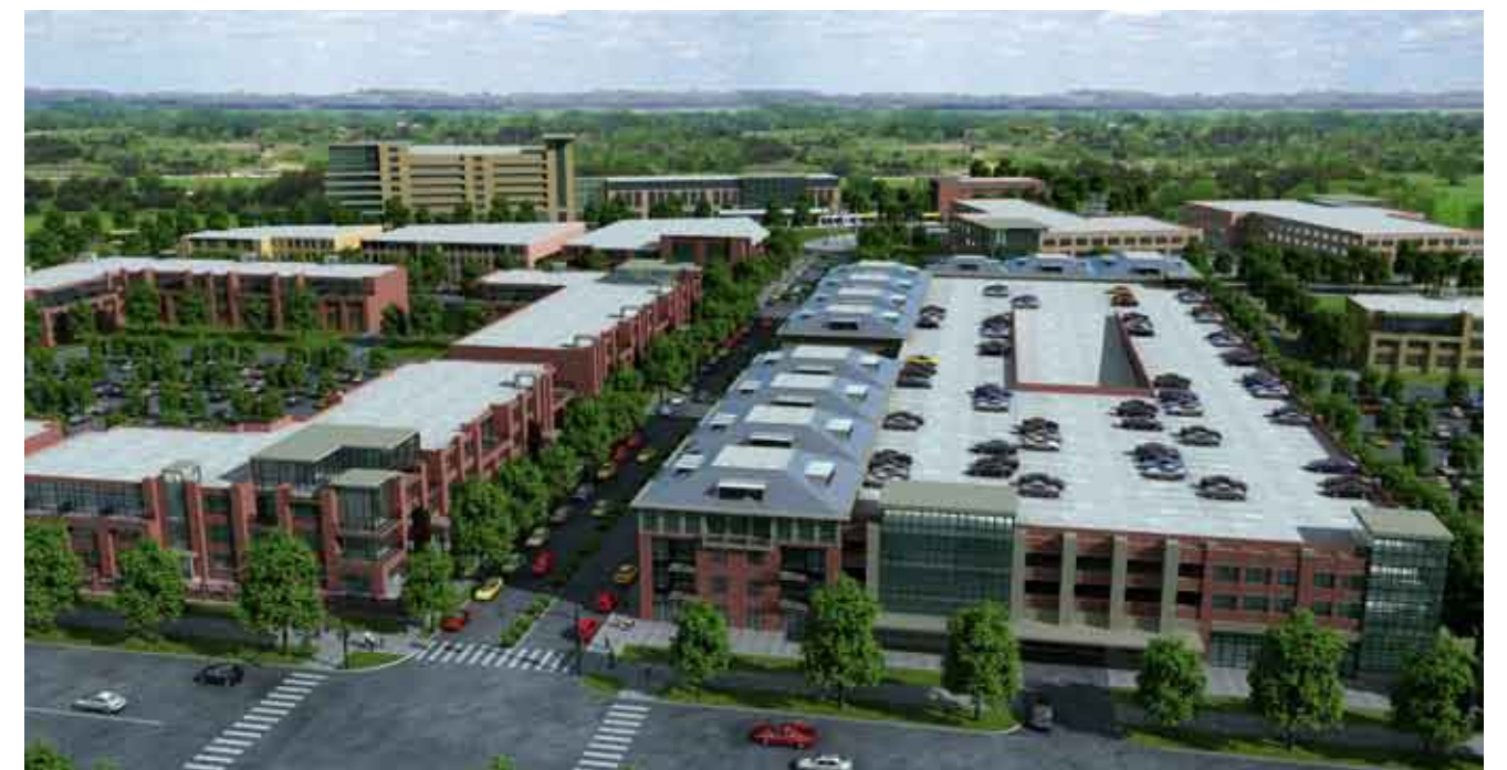
RENDERING LOOKING FROM EXCELSIOR BLVD DOWN THE NEW 17TH ST EXTENSION TOWARDS THE SHADY OAK STATION.
