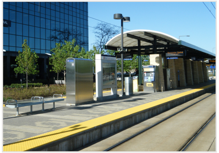
Station platform with shelter, signage, lighting, and seating
