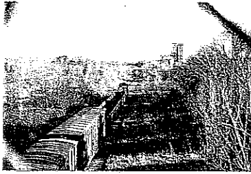
Minneapolis Northwest Corridor – Existing rail operations to be maintained.
