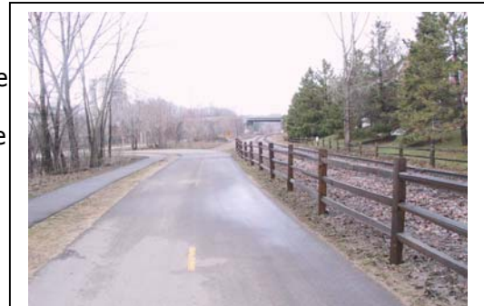
Trail and Freight Rail, Kenilworth Corridor
