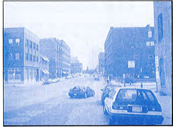
2nd Street Looking Southeast Across 3rd Avenue
