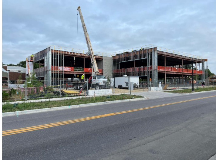
Pictured left: Second floor of north addition, ready for wall partitions and mechanical/electrical rough-ins. This building will house additional NorthPoint services.
