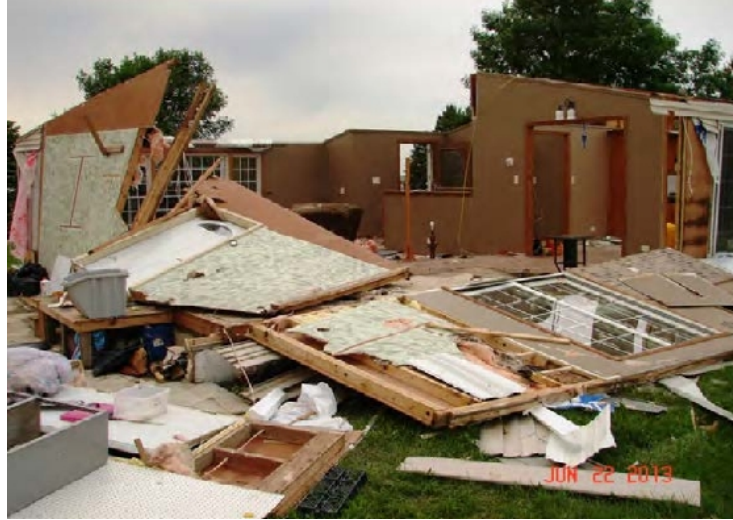
Figure 13. Extreme wind damage to Lake Poinsett cabin, courtesy of NWS Aberdeen. iii
