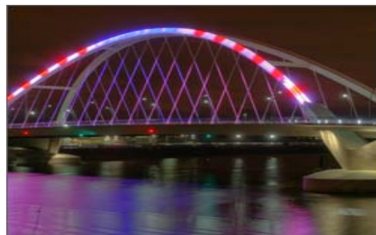
Lowry Avenue Bridge
