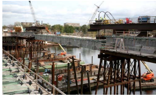
Lowry Avenue Bridge Construction
