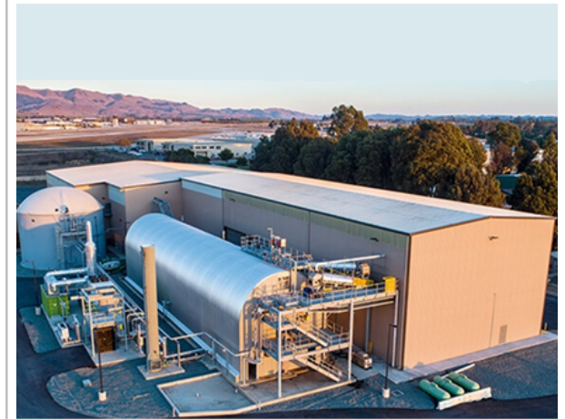
Anearobic Digestion Facility in San Luis Obispo, California
