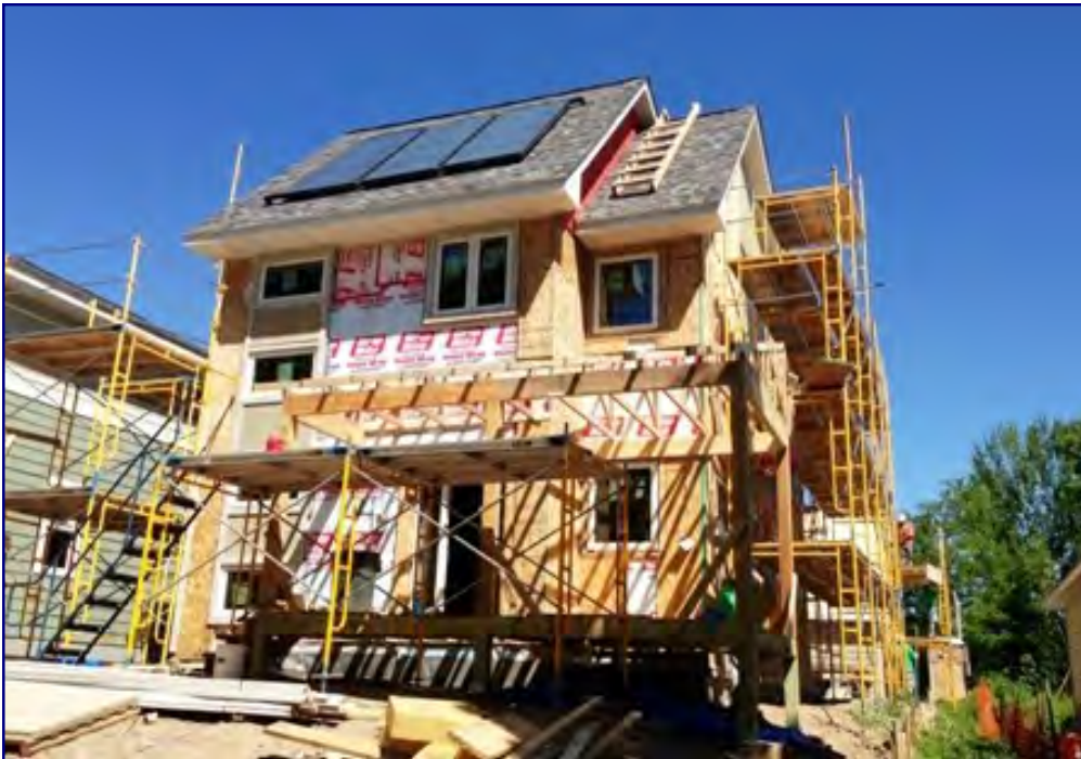
Above: A Green Homes North home under construction.
