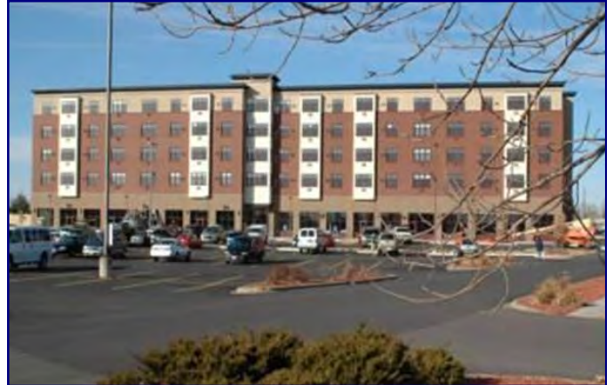
Above: Hiawatha Commons, located in Minneapolis near the Hiawatha Light Rail line.
