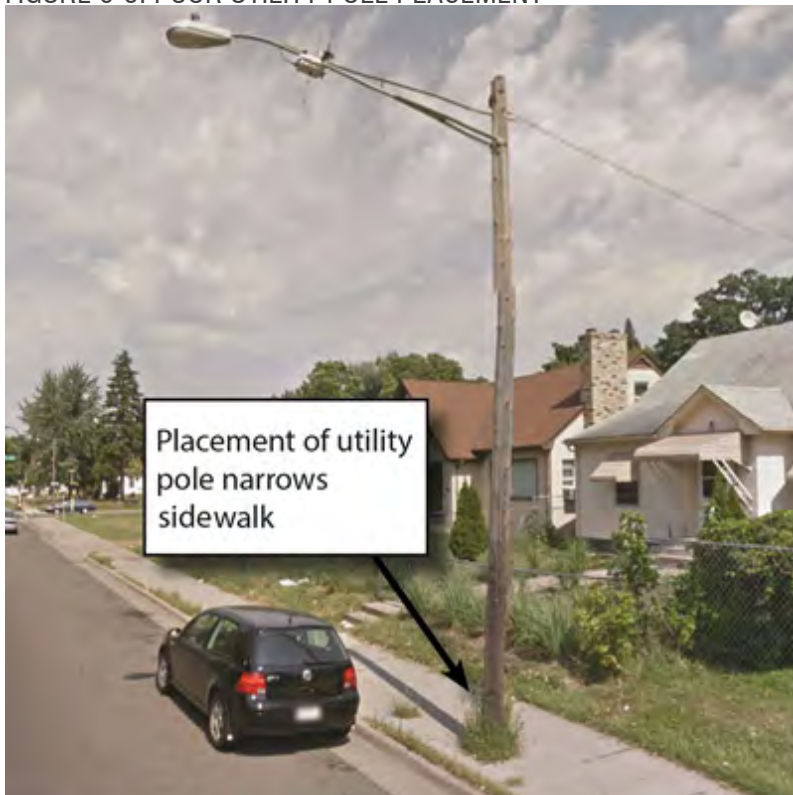
FIGURE 6-5: POOR UTILITY POLE PLACEMENT
