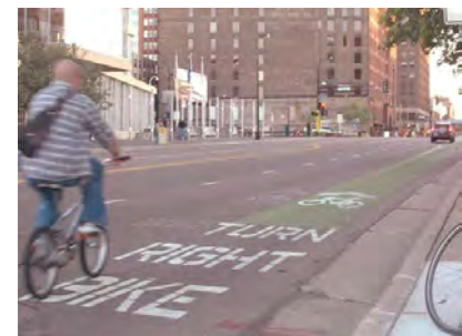
The Hennepin Avenue shared bicycle-bus lane: Buses, bikes, and right-turning cars share the right-most lane of travel. The green -striped “advisory lane” shows bicyclists where to ride so they are more visible to motorists, but cyclists are not required to ride in this area.
