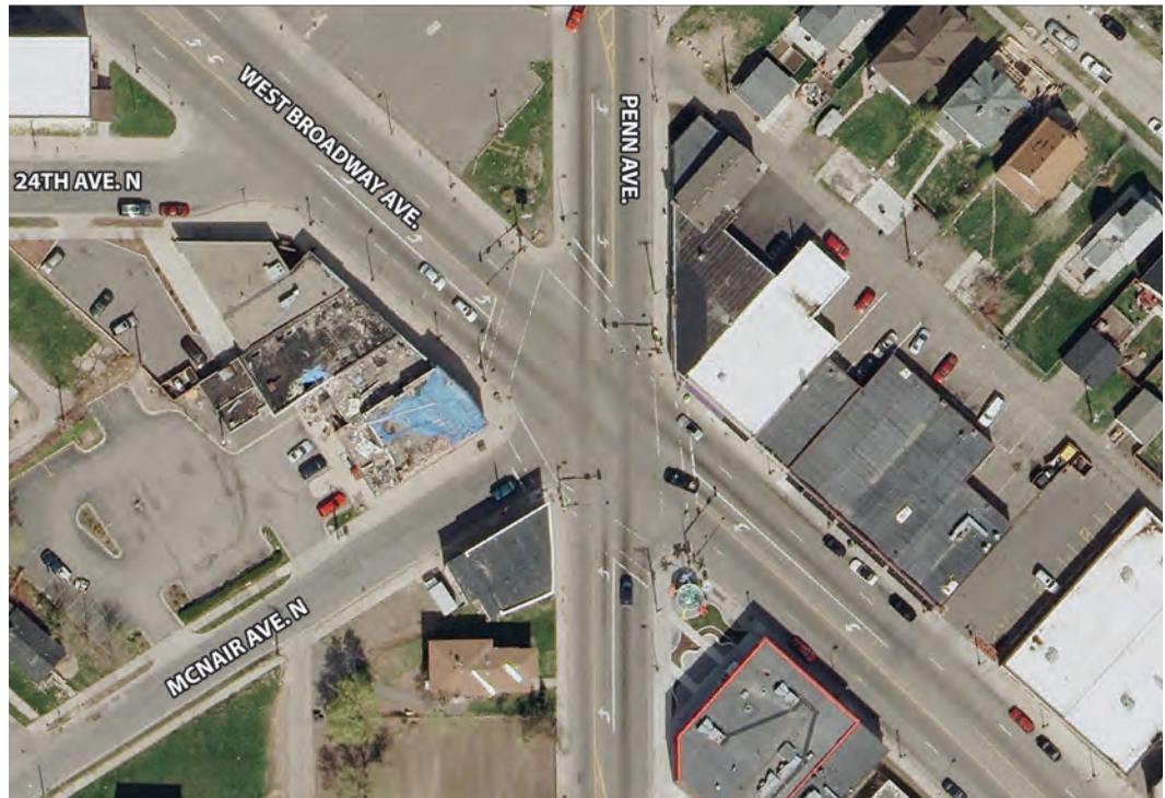
FIGURE 6-6: INTERSECTION OF PENN AVENUE AND WEST BROADWAY
