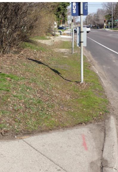
Sidewalk gap and obstructions along Crystal Lake Cemetery and Penn Avenue
