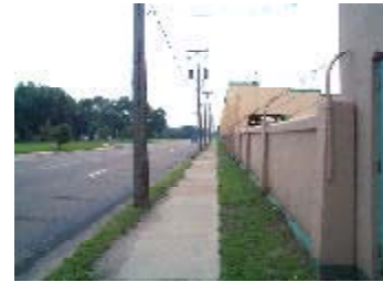
Reach 4 Lowry Ave. to 31st Ave. NE
