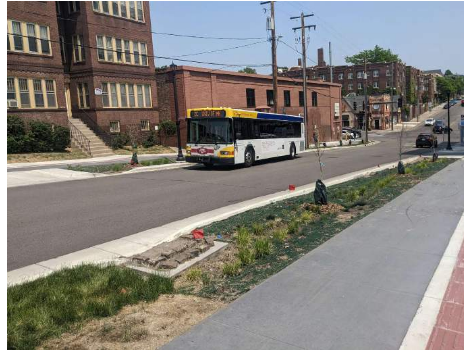
Stormwater management with new trees
