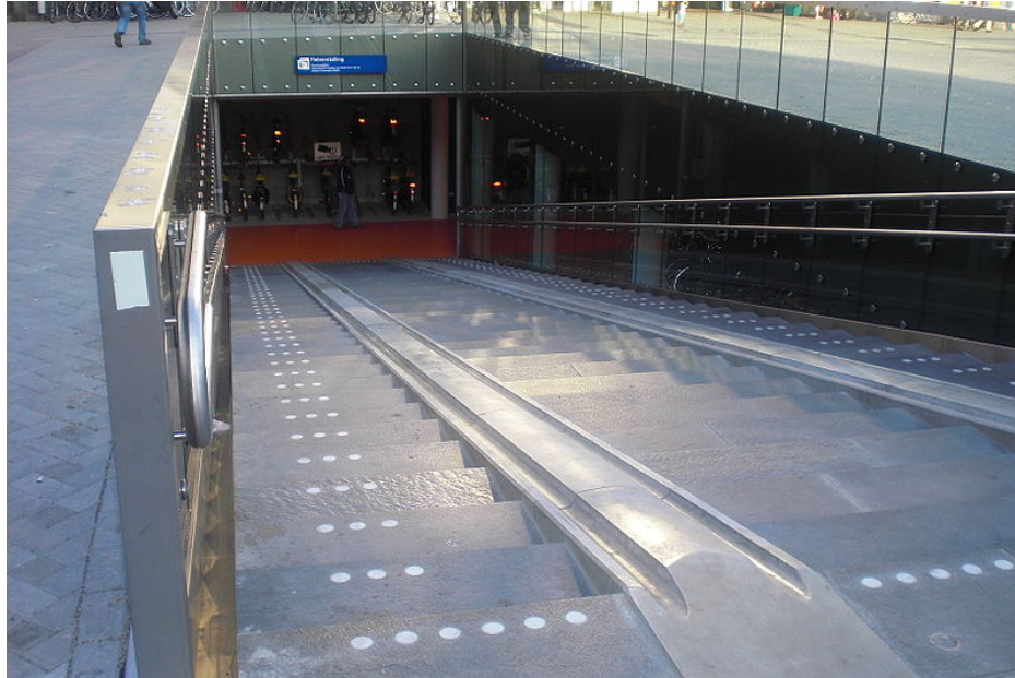
Figure 25. Dutch transit access stairway with bicycle channel
