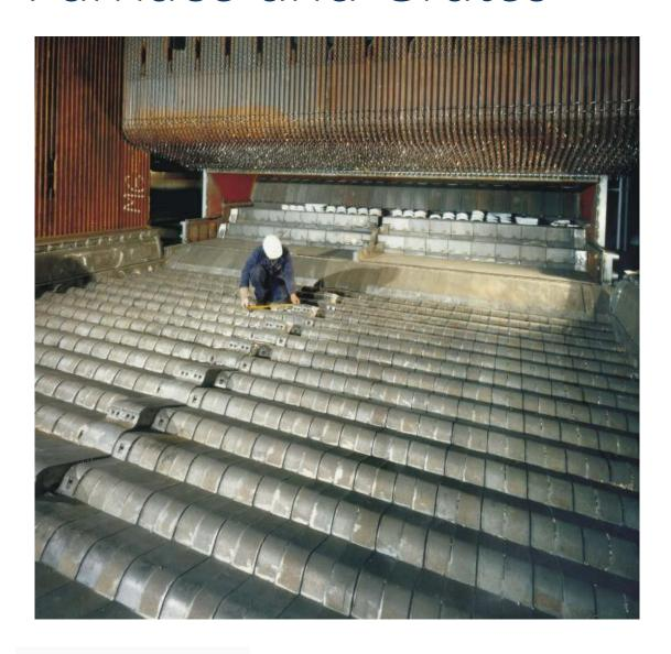
Furnace walls & ceiling are steel tubes filled with water.
