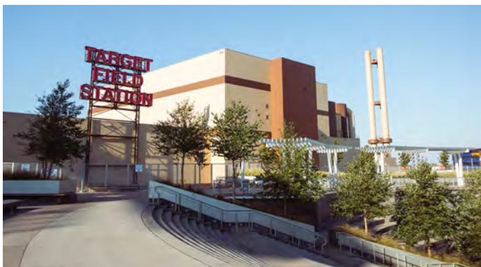
The Hennepin Energy Recovery Center (HERC) in downtown Minneapolis.
