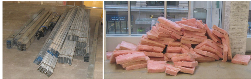
Salvaged metal studs and recovered batt insulation, ready for re-installation. Photos Stahl Construction
