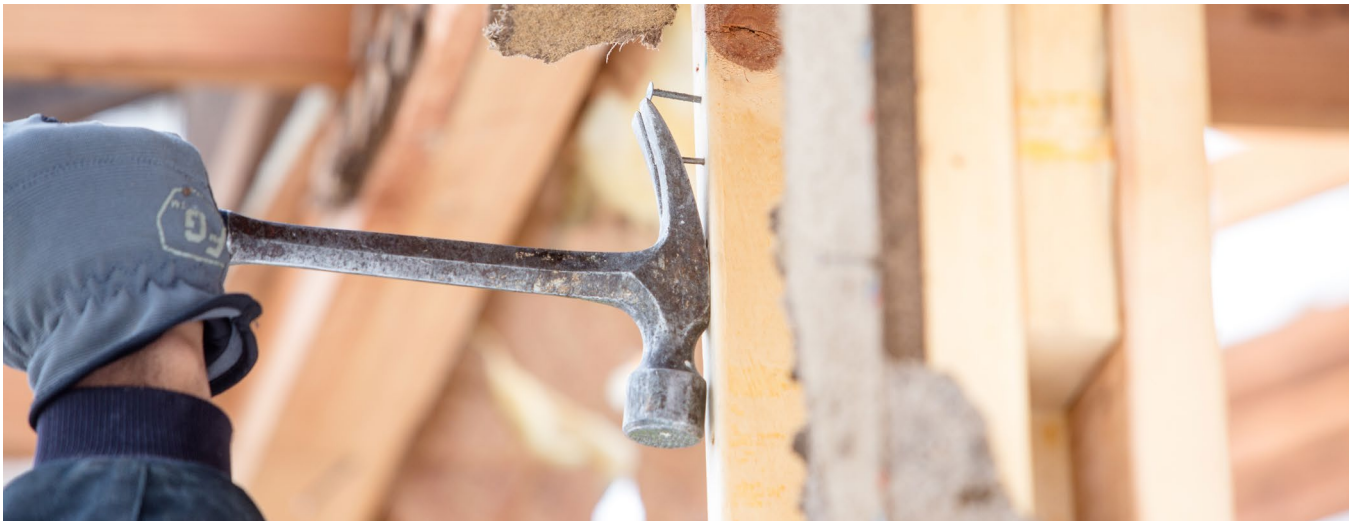
De-nailing a wood stud. Photo Hennepin County Energy & Environment
