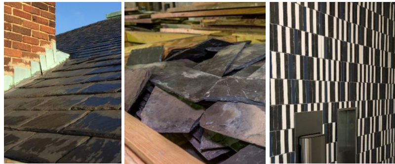
Slate tiles taken from a roof renovation and repurposed into restroom wall tile. Photos Lifecycle Building Center
