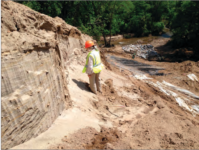
Figure 6.1 — Terrace Sand and Gravel Deposits
