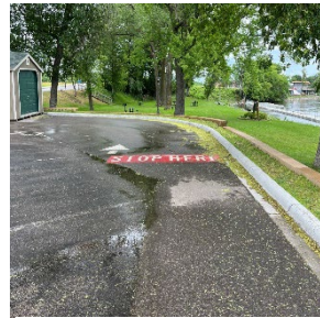
Image of Stop Bar near CD3 station
