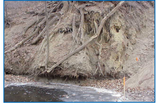
Example of soil erosion along a creek.
